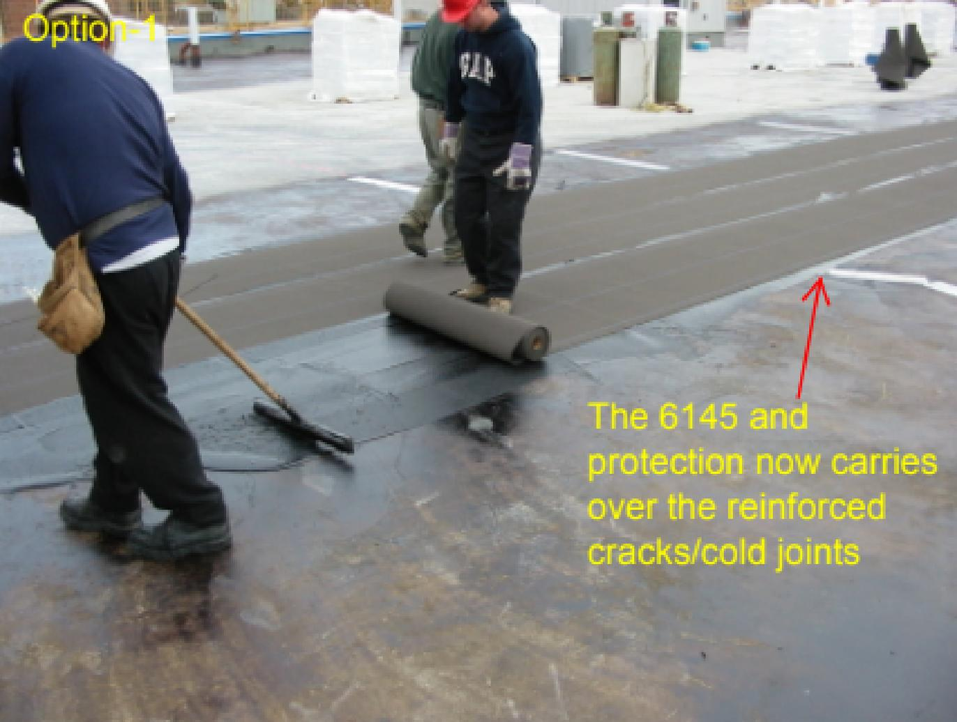
The 6145 and protection now carries over the reinforced cracks/cold joints
