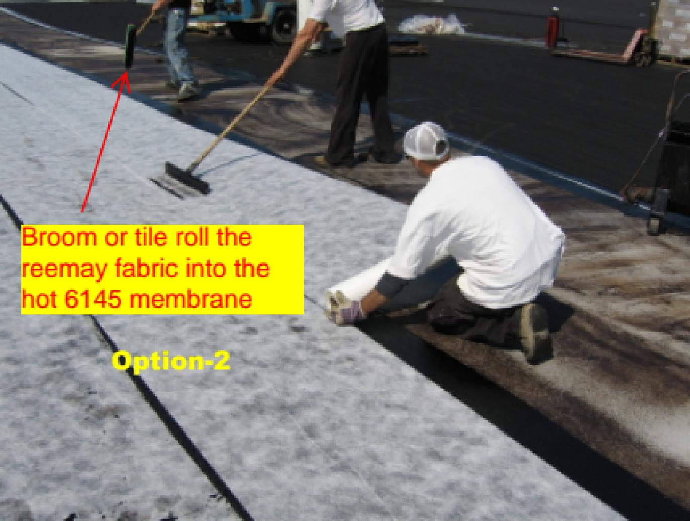
Broom or tile roll the reemay fabric into the hot 6145 membrane
