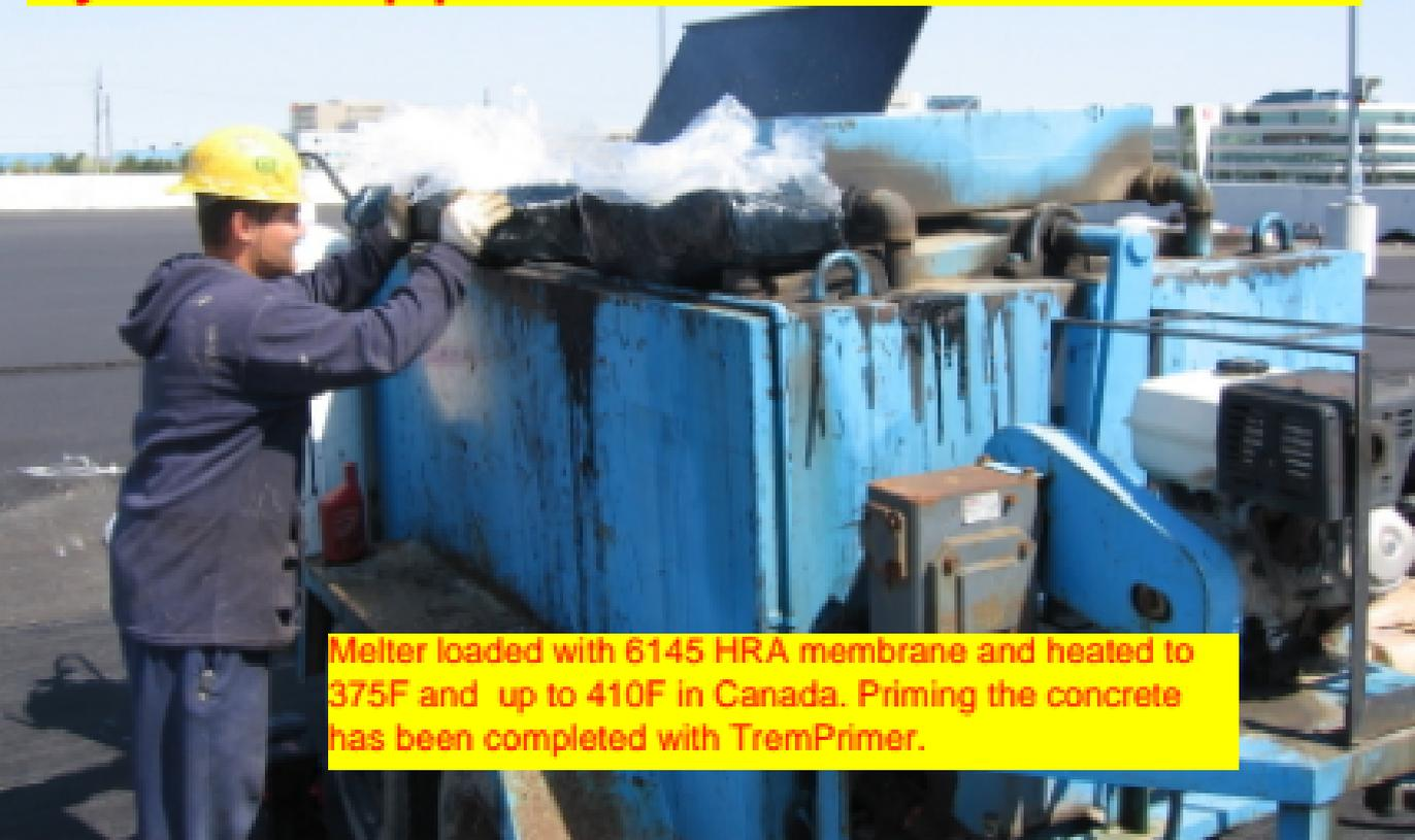
Melter loaded with 6145 HRA membrane and heated to 375F and up to 410F in Canada. Priming the concrete has been completed with TremPrimer.
