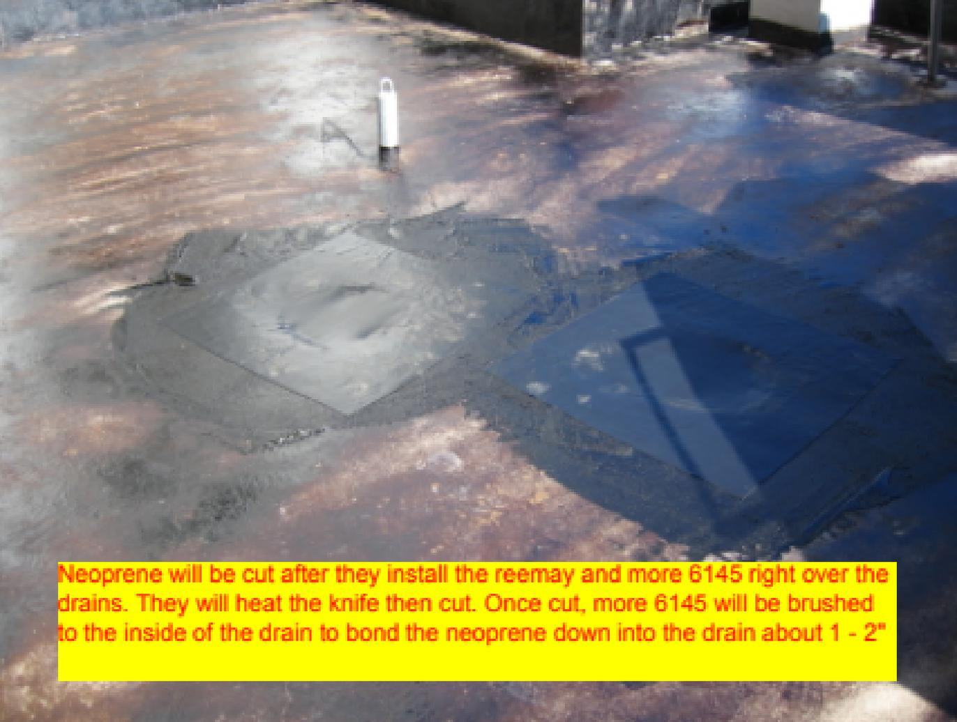
Neoprene will be cut after they install the reemay and more 6145 right over the drains. They will heat the knife then cut. Once cut, more 6145 will be brushed to the inside of the drain to bond the neoprene down into the drain about 1 - 2"
