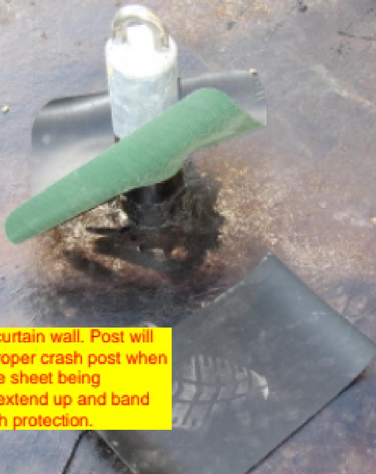
Parking deck over curtain wall. Post will be capped with a proper crash post when complete. Neoprene sheet being prepared. 6145 will extend up and band clamped to post with protection.
