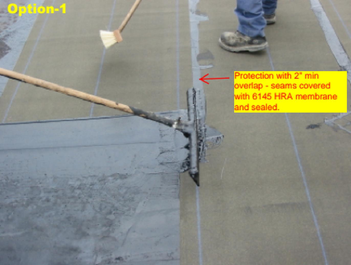
Protection with 2" min overlap - seams covered with 6145 HRA membrane and sealed.
